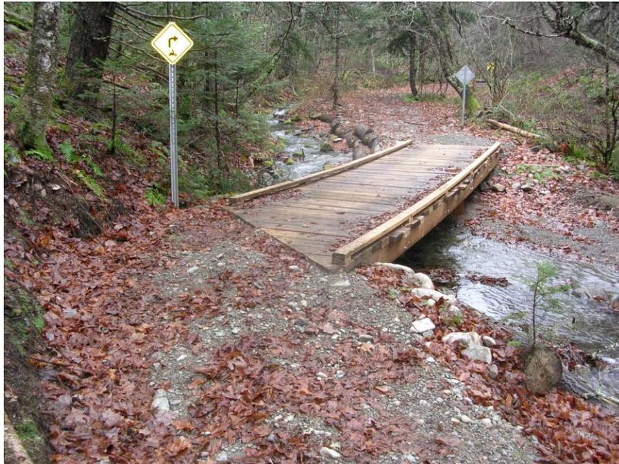
*Photo 4: The bridge in Turkey Hollow keeps ATVs from travelling 15m down the stream to cross the creek and the cribbing keeps high water flows from exiting the channel onto the trail, creating a win-win.*
